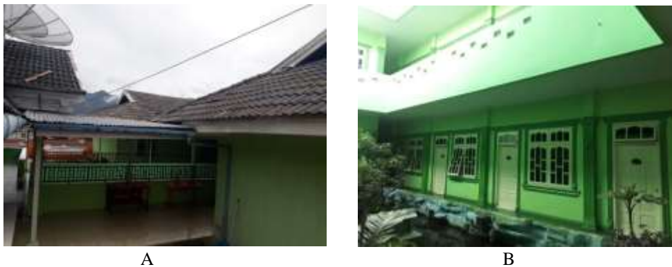
Figure 3. Condition of utility and fire protection. A. Lack of lightning protection facilities. B. Lack of fire-fighting sprinkler facilities
