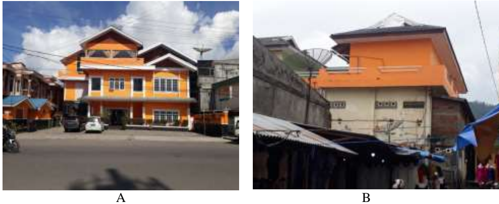
Figure 2. A. Overall architectural reliability condition. B. Architectural damage conditions
