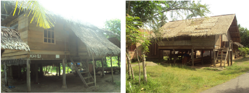
Fig.1. (a) Rumoh Aceh use timber/wood material; (b) Rumoh Aceh use sago palm and bamboo materials
