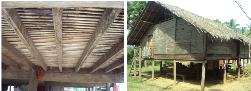
Fig.2.(a) Midrib of Sago Palm as wall's material; (b) Space between material
