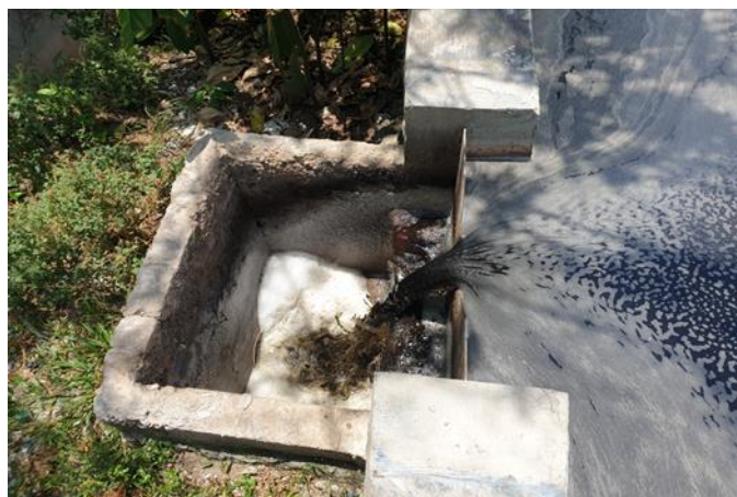
Figure 2. Leachate wastewater from the last pond of TPST Piyungan
